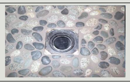
Completed drain connection with waste pipe slightly below no caulk compression nut.
