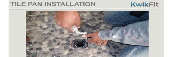
Install rubber gasket and caulking nut hand tight and then ¼ turn with key.
